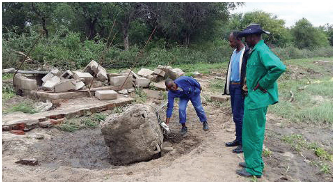
Following the incessant rains in the Mangwe district of the Matabeleland South Province, floods hit a thriving Makwakwa Irrigation Project supported by World Vision, damaging infrastructure worth around US$25,000.
